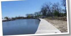
north side of the Dock A access road approximately 2 feet high and 14 feet wide to prevent wave surges that may go around the revetment.
